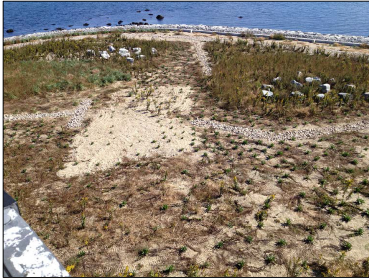
Figure 3: Cobble-filled drainage ditches on Bird Island and material excavated from the ditches used to raise elevation of a low spot (which appears mostly unvegetated) on the eastern section of the island, 17 October 2017. (Photo Credit: C. Mostello/MassWildlife)
