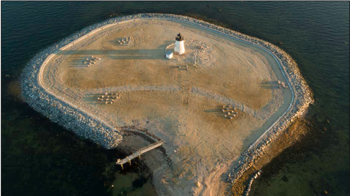
Figure 1: Bird Island on 11 April 2017, post-construction. (Photo Credit: M. Moore.)
