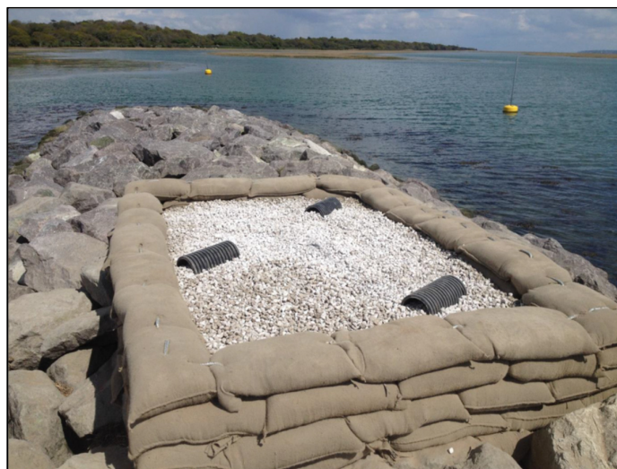
Figure 1: Breakwater bunds ©Daniel Piec
