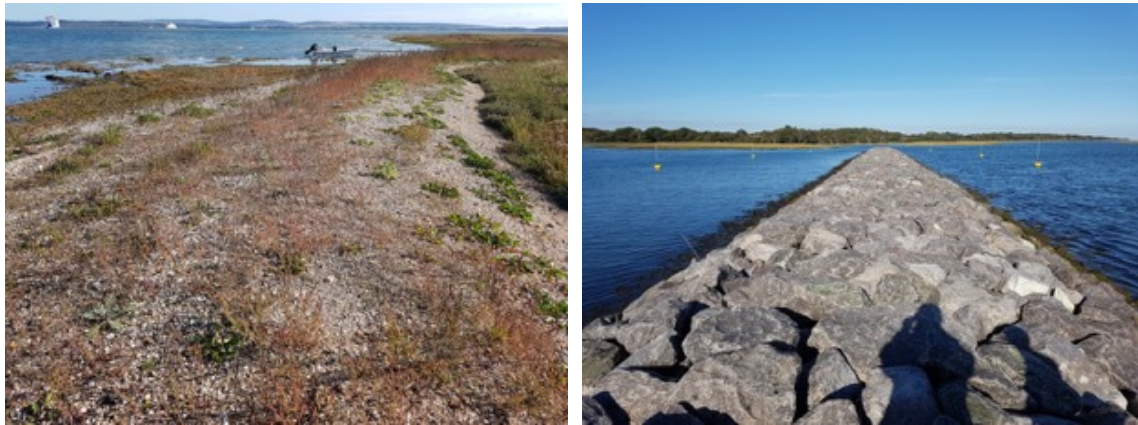
Figure 3. Shingle recharge area and breakwater for the installation of nesting platforms in Solent and Southampton Water SPA in south England.
