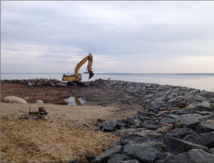
Figure 26: Construction of the new revetment on Bird Island, December 2016 © C. Mostello/MassWildlife
