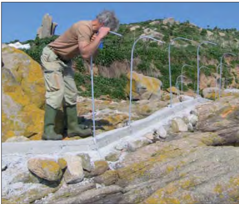
[6] Top left: the team of volunteers after digging the trench on the Isle aux Dames on 11 March 2009. [7] Top right: transportation by helicopter proved to be the most appropriate method to carry the 24 tons of materials between the mainland and the Isle aux Dames. [8] Down left: the removable metal posts supporting the wire fencing are secured to the concrete base. [9] Down right: an electrified wire gate supplied by a solar panel is attached to the bent edge of the wire fencing. A gate provides access to the colony for biological monitoring (count, ringing...).
