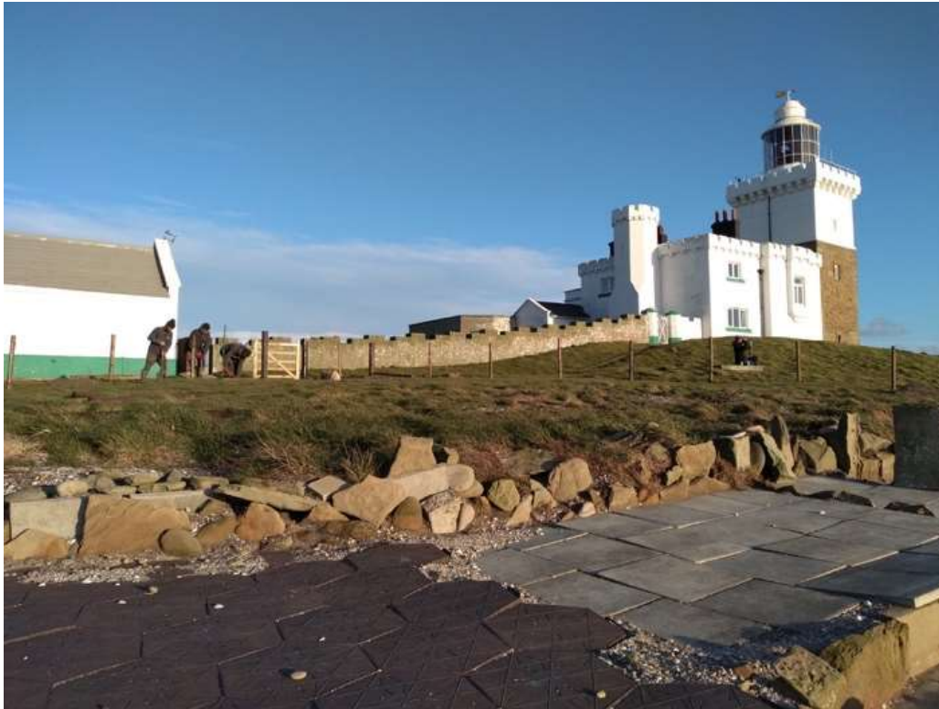
Figure 16: Construction of the South terrace fence
