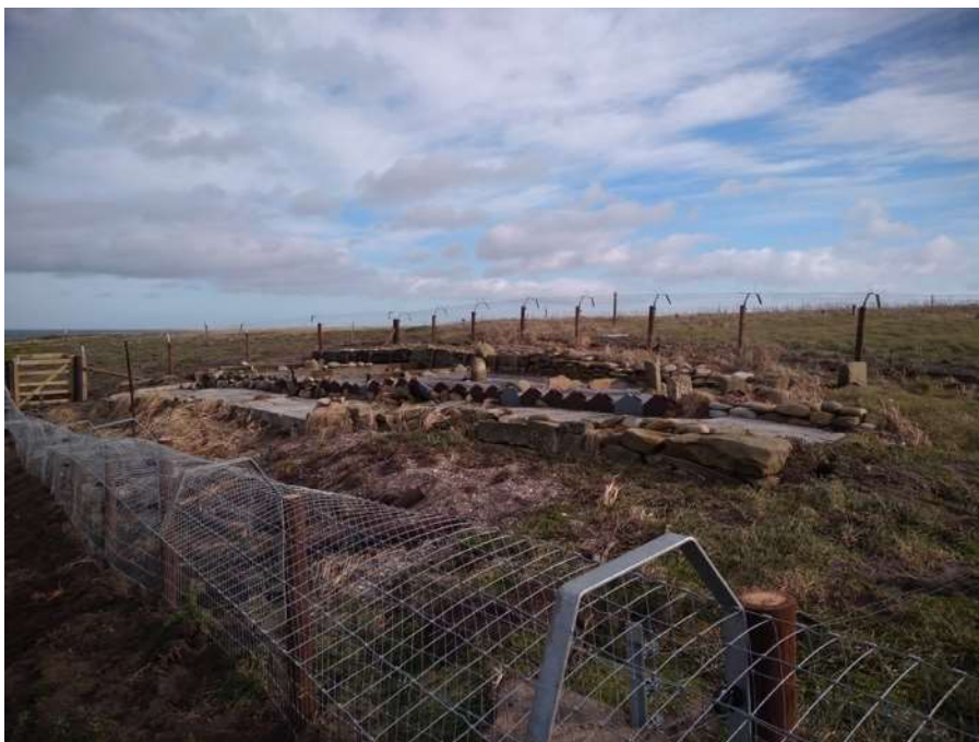
Figure 15: Construction of the North terrace fence
